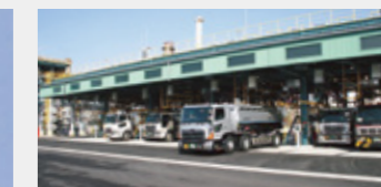
Shikoku Operations Lorry loading facilities
