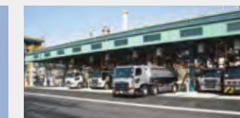
Shikoku Operations Lorry loading facilities
