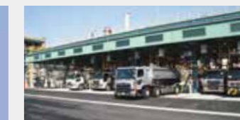
Shikoku Operations Lorry loading facilities
