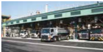
Shikoku Operations Lorry loading facilities
