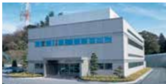
Shikoku Operations Lab Center
