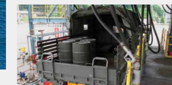
Shikoku Operations Drum distribution facilities
