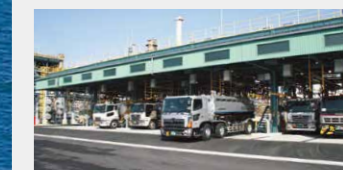
Shikoku Operations Lolly loading facilities
