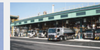
Shikoku Operations Lorry loading facilities
