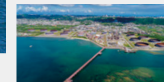
Nansei Sekiyu K.K. (Nishihara-cho, Okinawa) Supplies petroleum products within Okinawa Prefecture via the Company's terminal.
