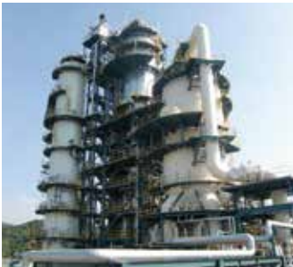
Resid fluid catalytic cracking unit
